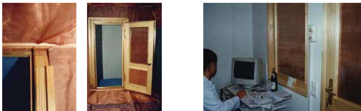
Room shielding to solve the requested electromagnetic compatibility
